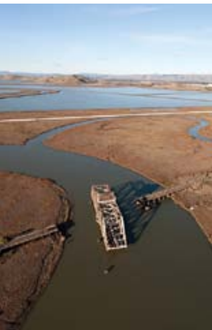
Dumbarton Cutoff Line —Newark Slough Swing Bridge
