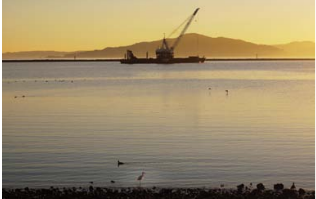
Dredge at sunset
